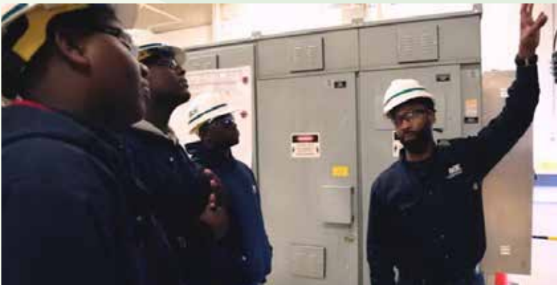
Jelani Wise, Dante Watkins and Keyon Brown —pictured listening intently to Sr. Training Specialist Frank Howell (right)—were hired as substation technician trainees after interning at BGE for two summers.
